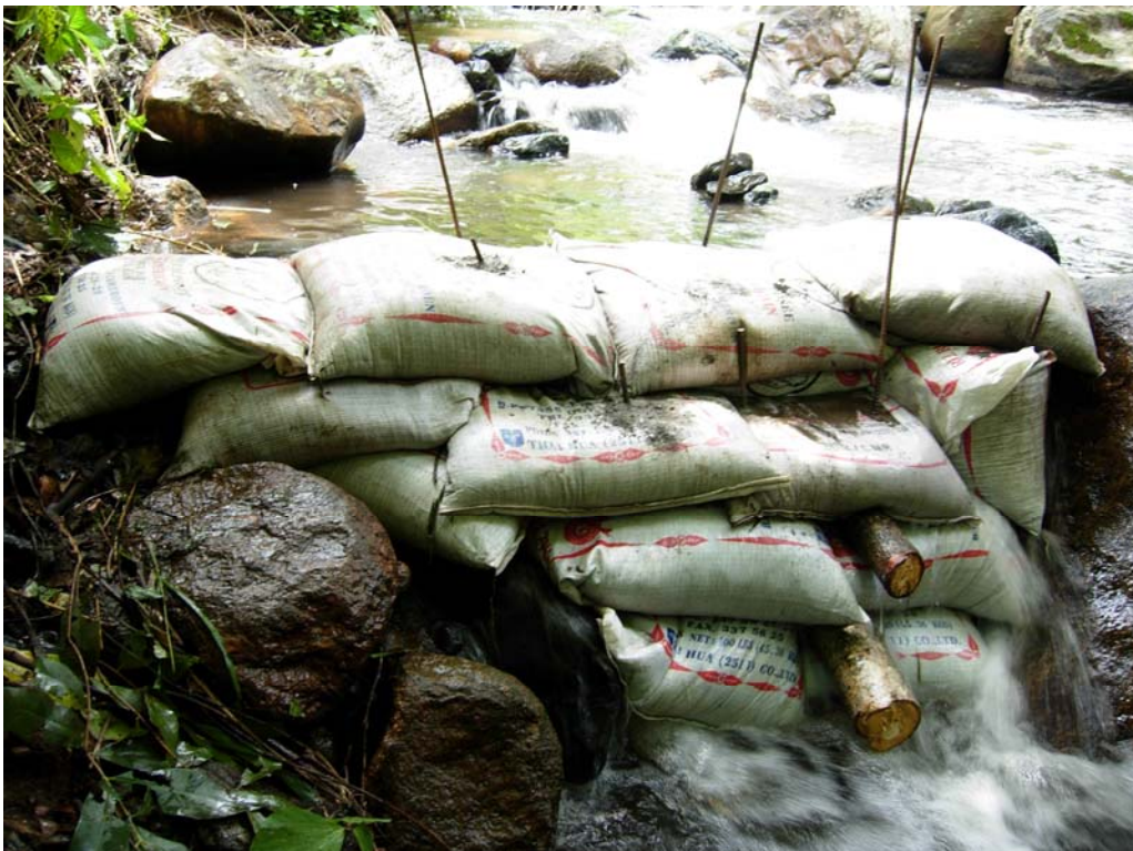
Figure 2: Photograph of preliminary dam constructed in May 2007.
