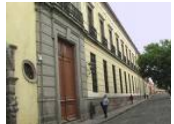
Educational building at the downtown UAQ campus
