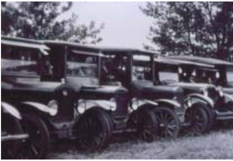
Autos lined up at Lakewood Farm, c. late-1920s
