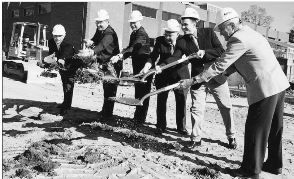
Work on the science center had started in March, but a ceremony on Thursday, May 2, provided an opportunity both to celebrate the occasion and to help along the construction team a bit. From left to right are: Dr. James M. Gentile, J. Kermit Campbell, President James E. Bultman '63, Dr. George Zuidema '49, Matthew Nehs '02 and Dr. Donald Mulder '48.
