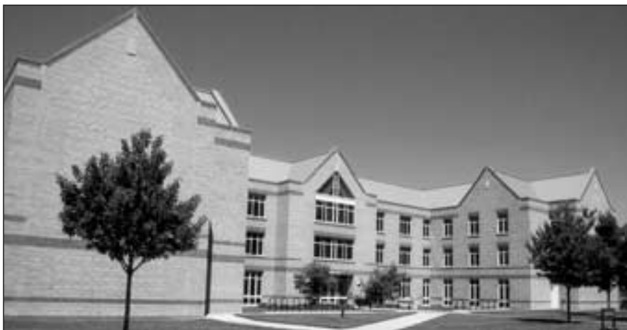
Construction is beginning on an addition to Cook Hall scheduled for completion by the start of classes in the fall of 2006.
