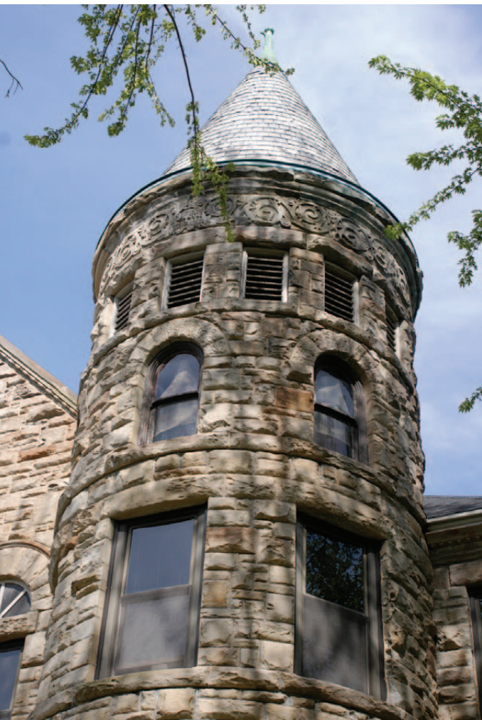
Firm Foundation. Hope builds on a strong past, literally as well as figuratively. The recent restoration of Graves Hall assures that the building will meet well the educational needs of the 21st century while celebrating Hope's history.
