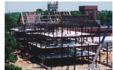
New Science Building under construction
