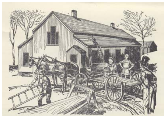
A building project in Holland
