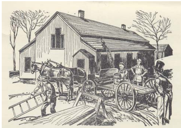
Construction in Holland
